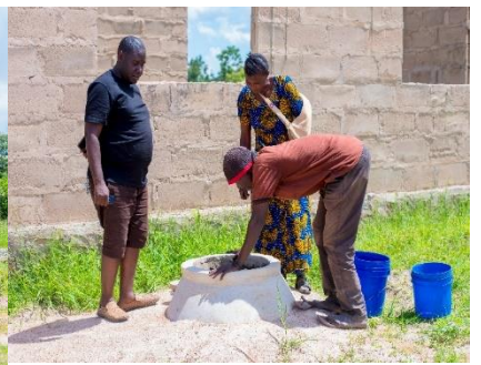
RAIN WATER HARVESTING TANK CONSTRUCTION
